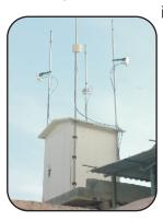
installed in the jails to rule out any possibility of use of mobile phones by the inmates in jails. There is a proposal to instal more jammers to the remaining jails during the year. These jammers block the communication in GSM 900/1800 MHZ and CDMA
